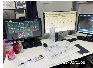
Graphic Annunciator Fire Alarm System
