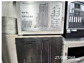
Graphic Annunciator Fire Alarm System
