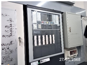
Fire Alarm Control Panel
